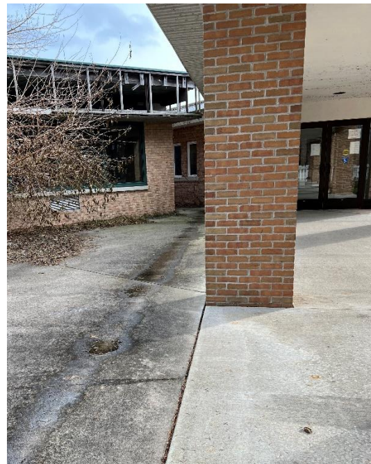
Remove concrete to left of expansion joint, preserve to the right
