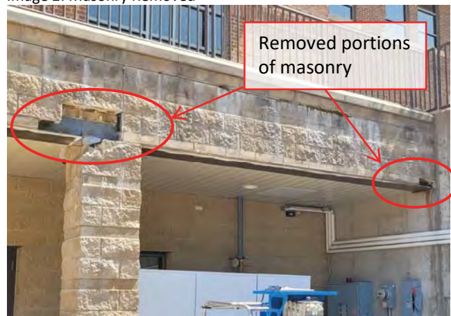
Image 2: Masonry Removed
