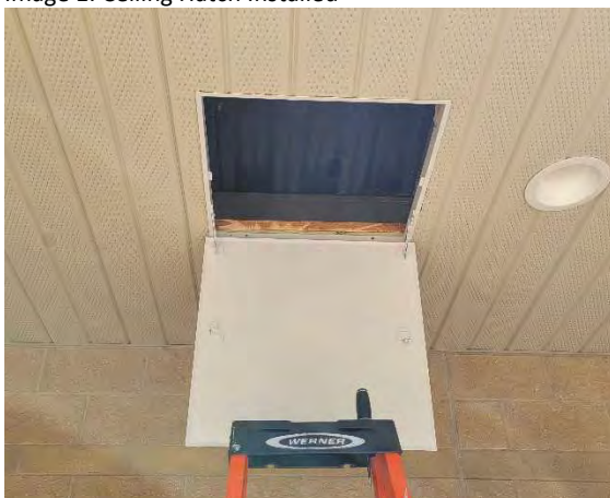
Image 1: Ceiling Hatch Installed
