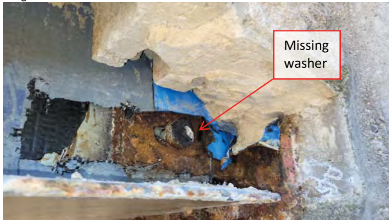
Image 6: Bolt without washer
