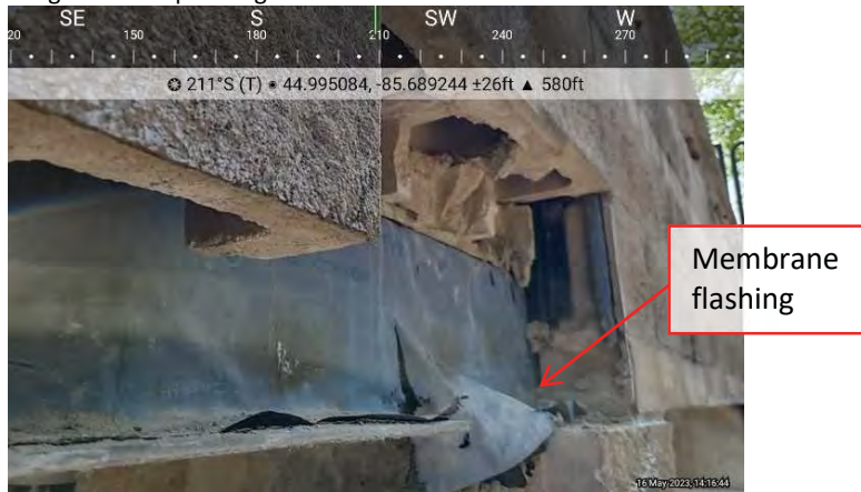
Image 3: Waterproofing over steel lintel
