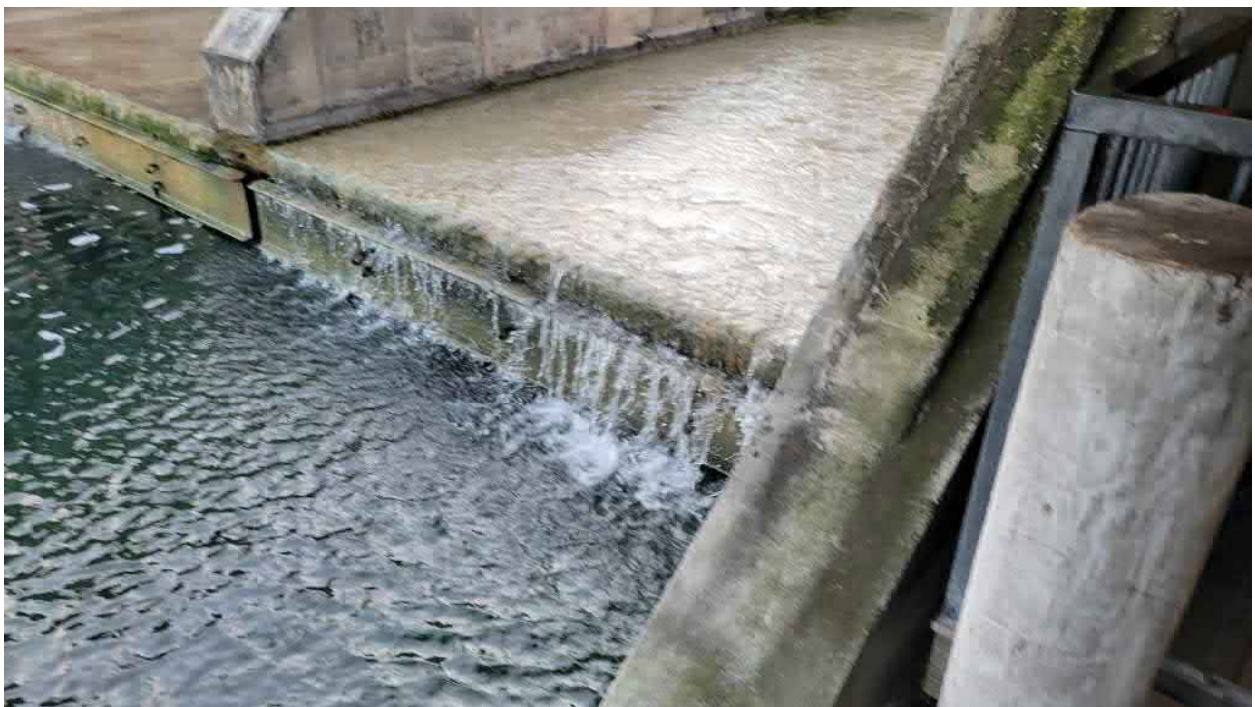
Downstream Face of Auxiliary Spillway
