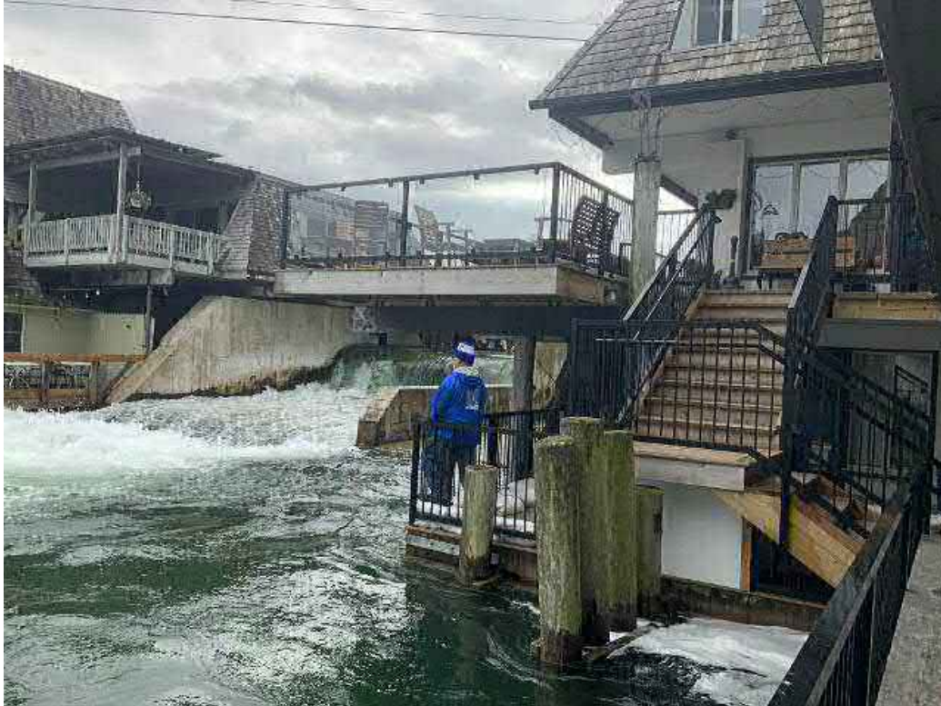
Looking east across at downstream side of dam.
