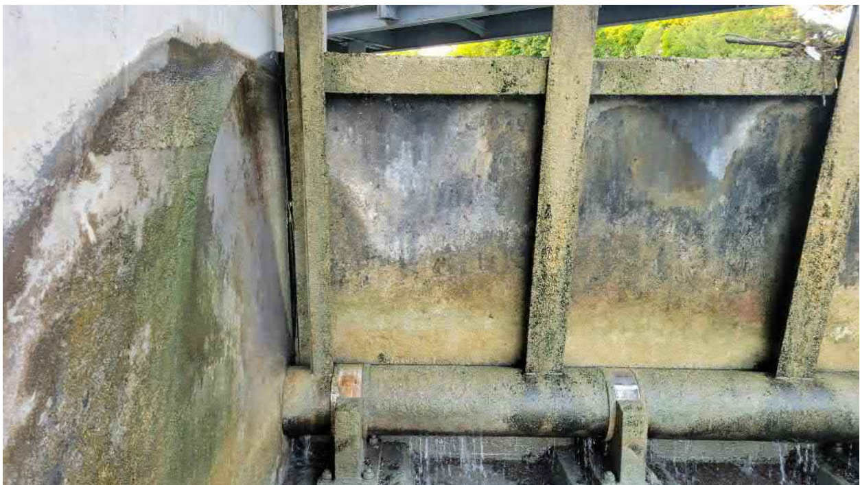
Gate Observations - Right Wall and Joints (Closed Position)
