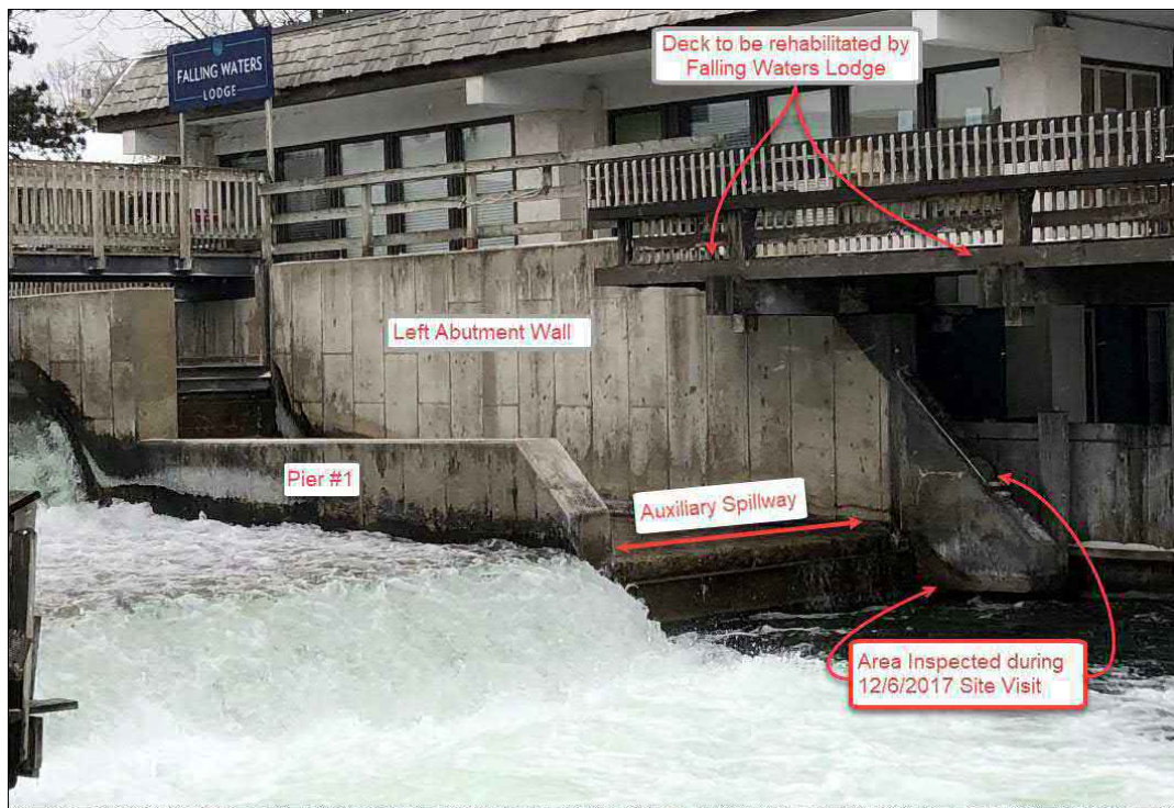
Looking South at Auxiliary Spillway, Left Abutment Wall
