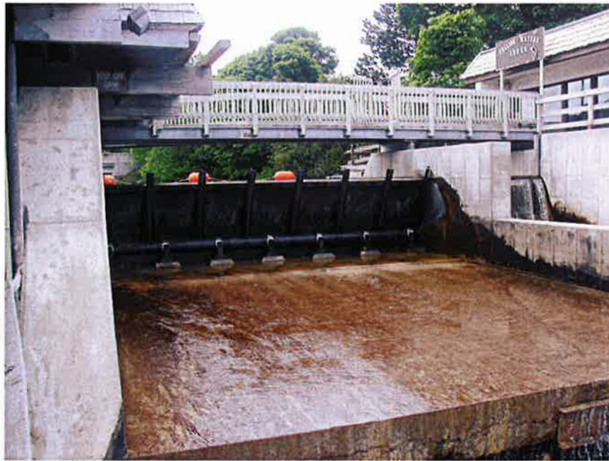
Photo 4. DS view of primary crest gate and operators/access bridge. Gate up.
