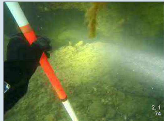
Pier #3 downstream end
