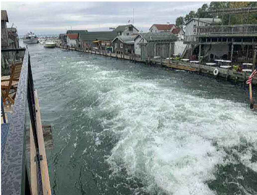
Looking northwest at downstream channel.
