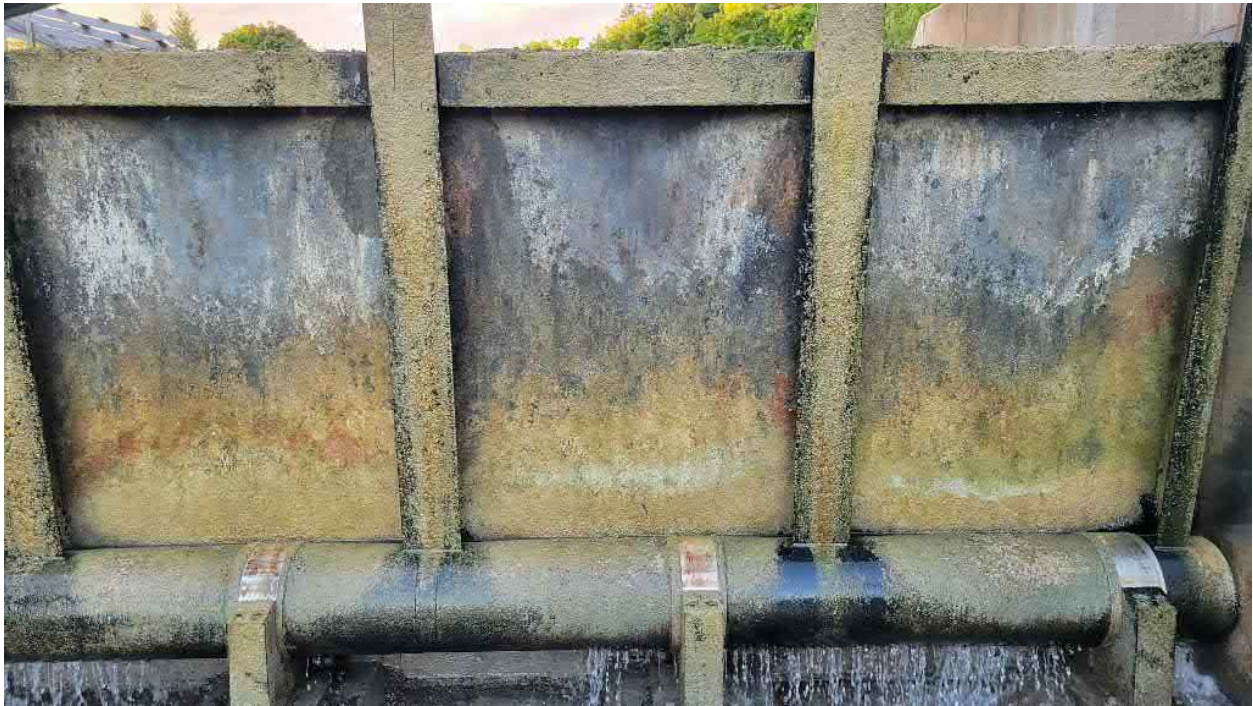
Gate Observations - Downstream Face (Closed Position)
