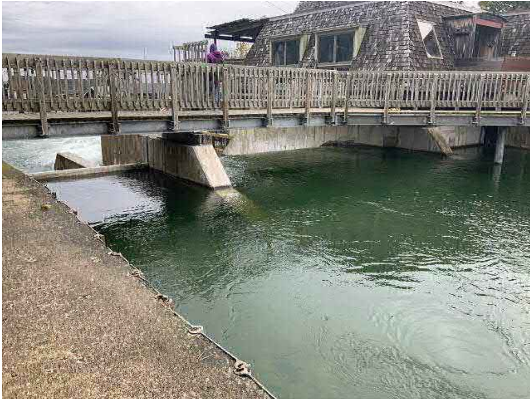
Looking north at walkway and upstream side of dam.
