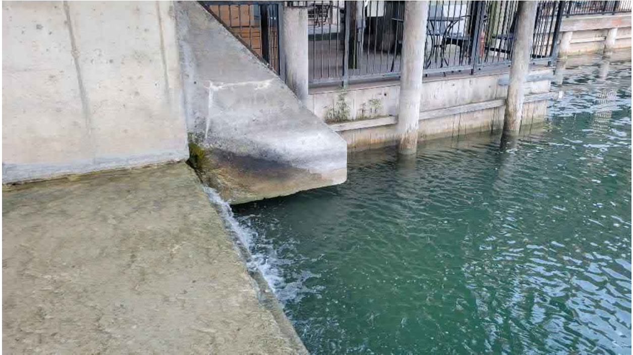
Right Abutment of Auxiliary Spillway
