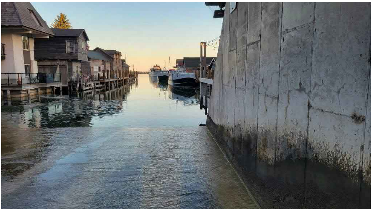
Right Wall of Primary Spillway
