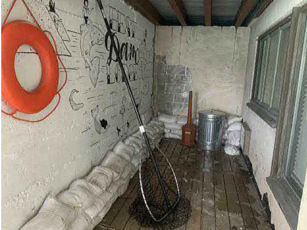
Looking southeast at outside of Bay #1 left abutment wall.
