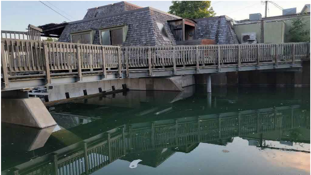
Catwalk above Dam to Access Auxiliary Spillway Boards
