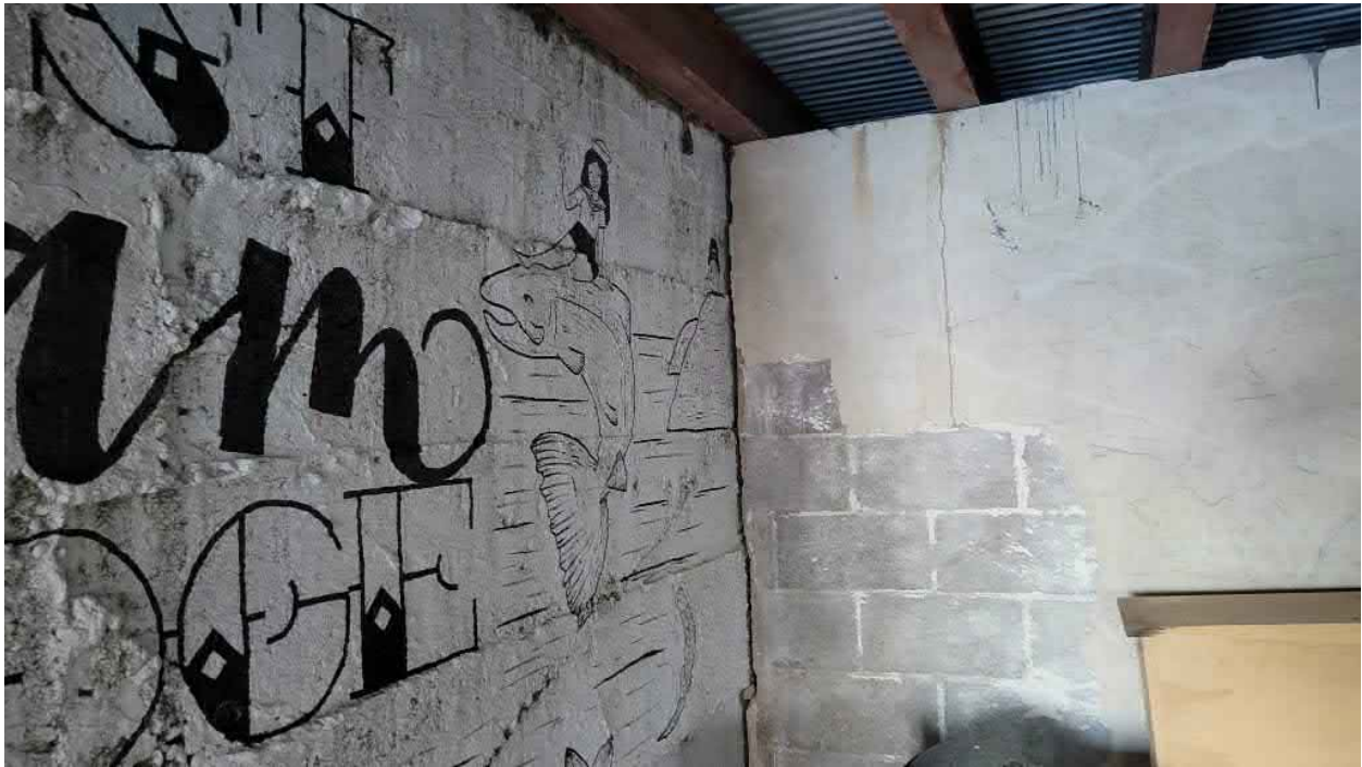
Left Abutment Wall and Wall Adjacent to Dam
