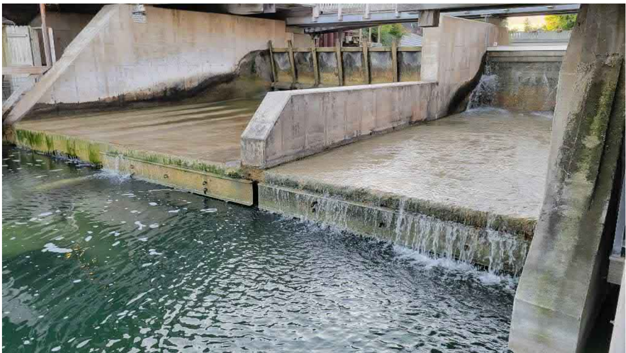
Downstream Face of Spillways
