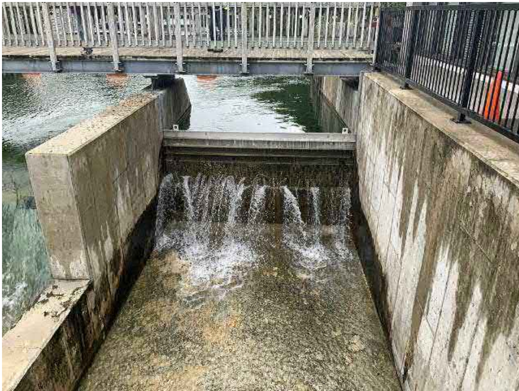
Looking southwast at Bay #1 (fixed concrete crest with removable aluminum stoplogs).
