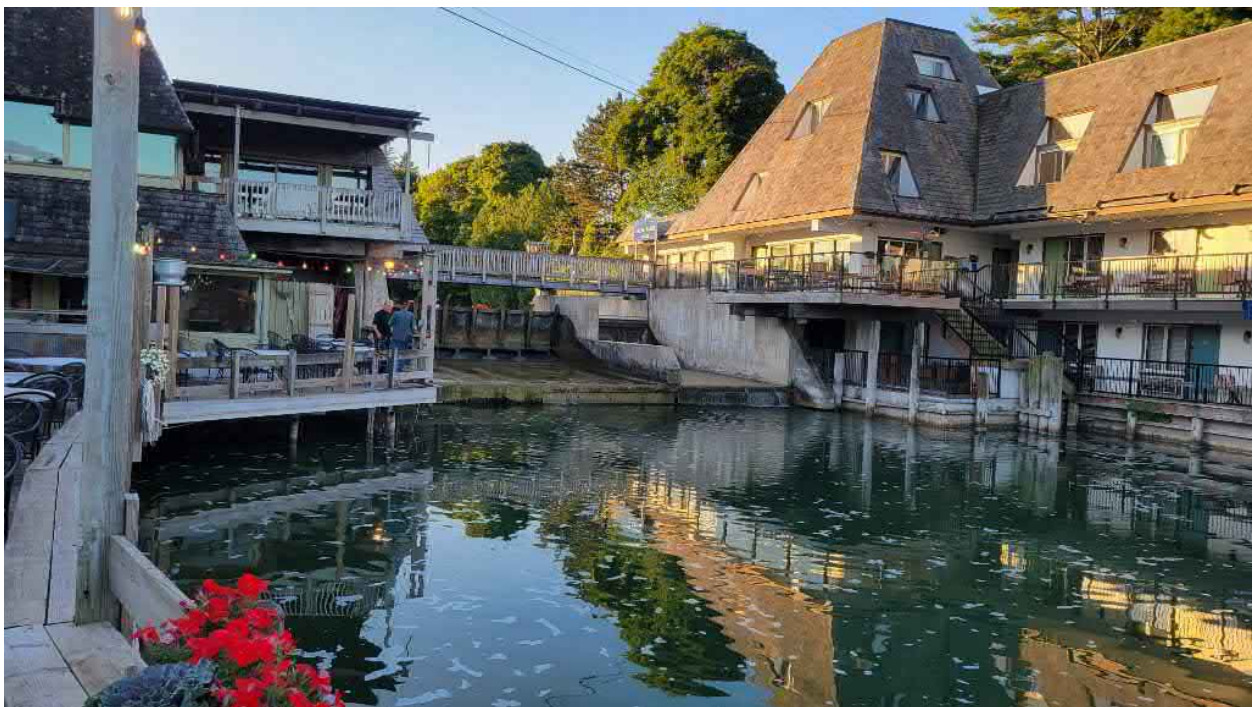
Downstream Face of Dam
