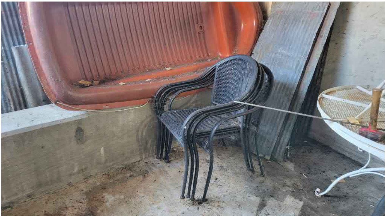
Control Room - Concrete Curb Flood Protection
