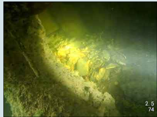
Left abutment (downstream end)
