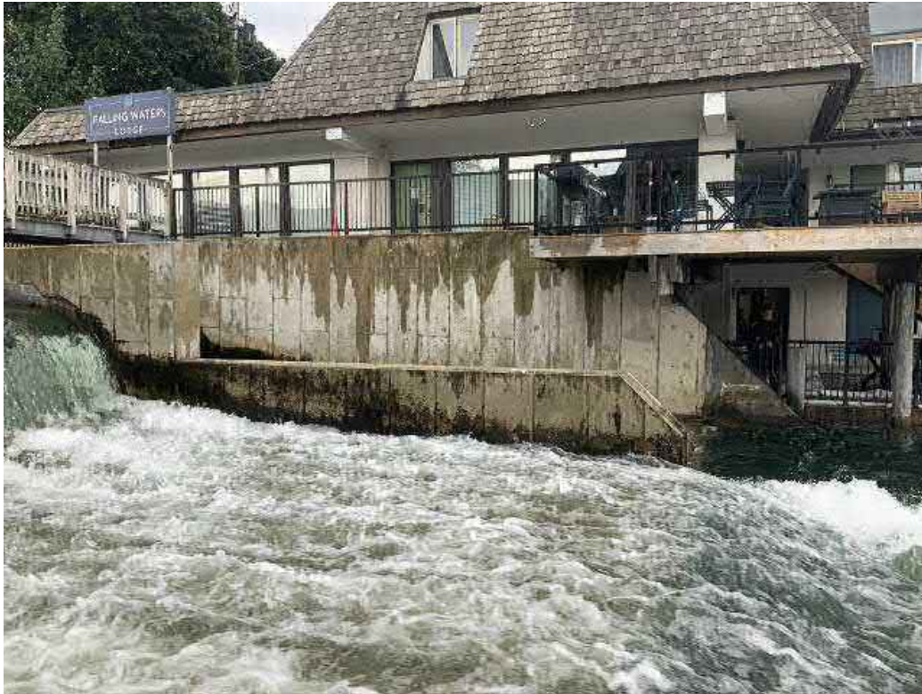
Looking south at principal spillway left abutment wall.
