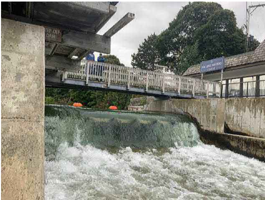
Looking southeast principal spillway (actuated weir gate).
