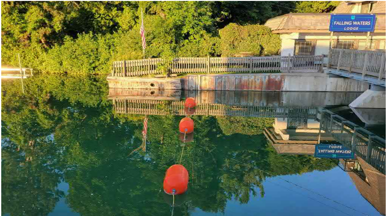
Upstream Buoys and Left Abutment Wall
