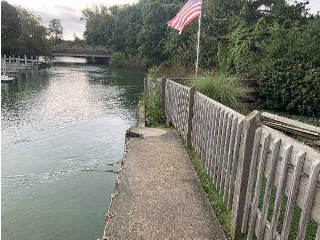
Looking southeast at upper end of left approach abutment wall and wooden seawall.
