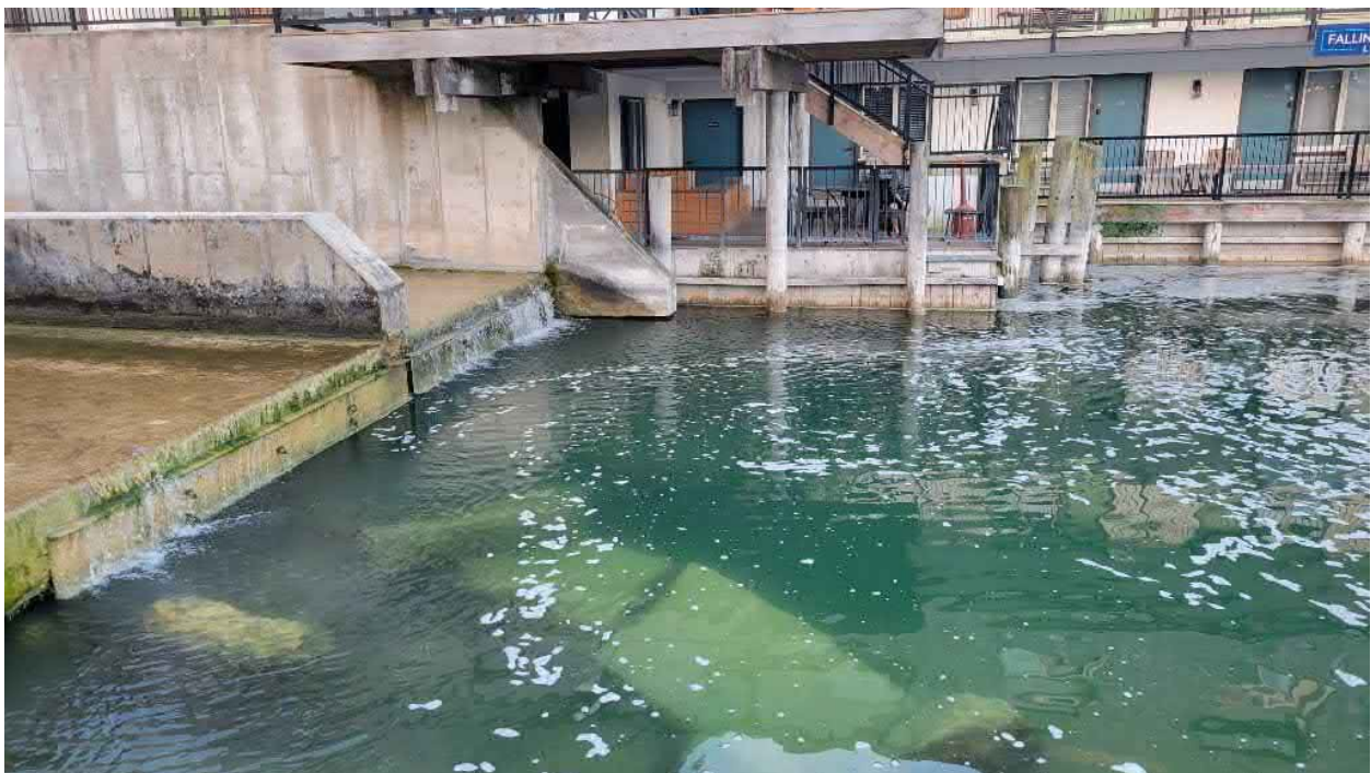
Spillway Observation While Gates are Closed
