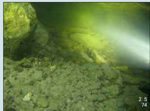
Cutoff wall and right abutment
