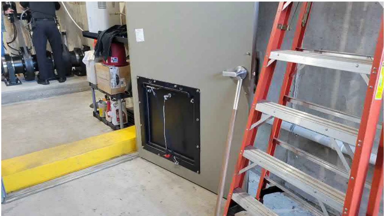
Control Room - Secondary Concrete Curb Flood Protection and Escape Hatch
