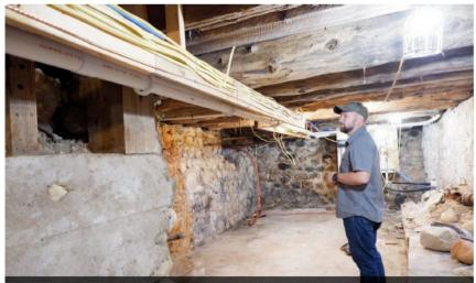
Picture of progress: all new electrical and plumbing, plus a new furnace and air conditioning have been installed. Many more structural improvements, too: there are new footings in the basement, and two new redesigned staircases. Above, Chase looks at the new electric & plumbing in the basement. Notice the original cectar beams from 1855, still with bark hanging off, above Chase.
