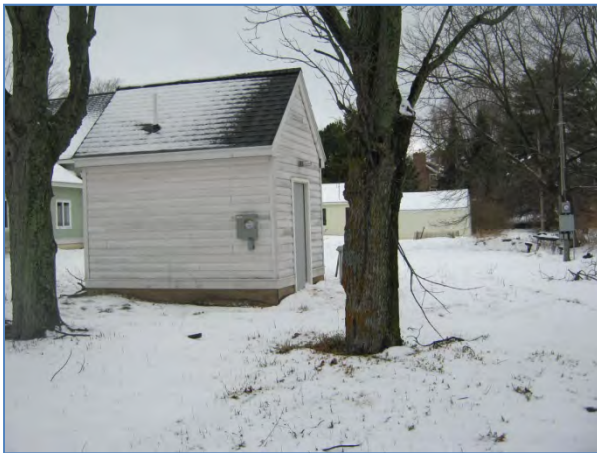
Completed Well House Viewing Easterly
