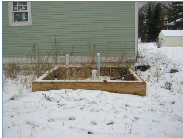
Incomplete Well House
