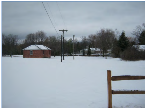
Unit #6 Viewing Westerly
