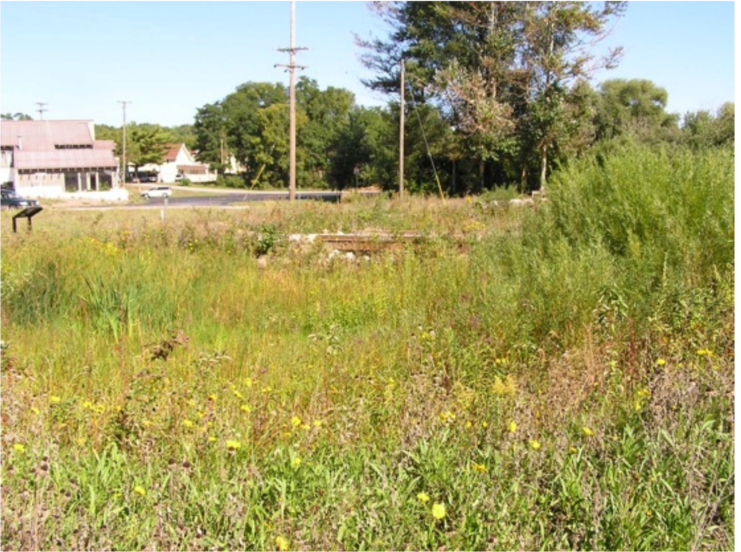
Year 2 - Shallow basin of the innovative stormwater treatment system, ISEA Center, 100 Dame St., Suttons Bay, MI - Grobbel Environmental & Planning Associates design and construction.
