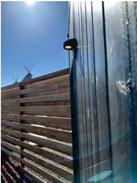
Figure 8 Staff Breakroom/Laundry Lighting
